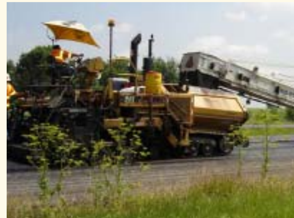
APAC-Missouri Inc. paves SRI project on Interstate 70.
